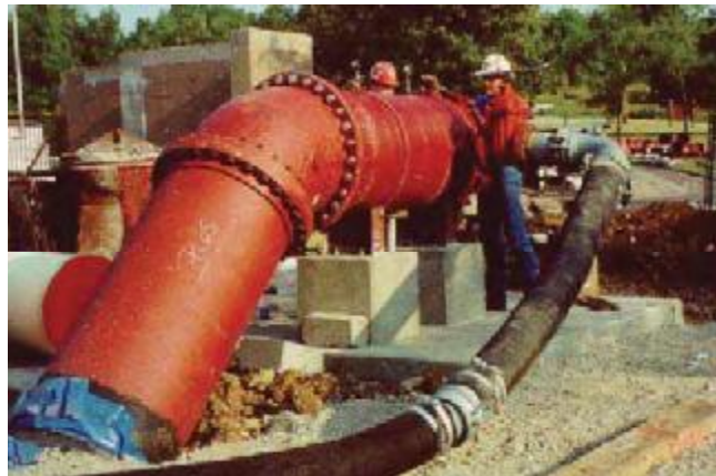
FIGURE 10.28 Original Photograph with Two Men and Pipe
