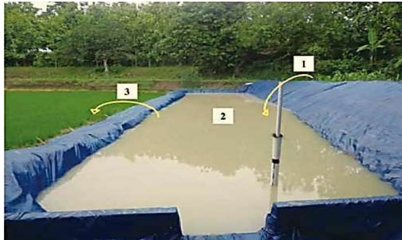
Figure 3. RWH using land surface for catchment area and reservoir for storing rain-off (Source: Mun, J. S., & Han, M. Y. (2012))
