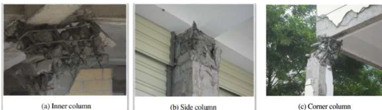
Figure 1: Column Failure at Various Locations
